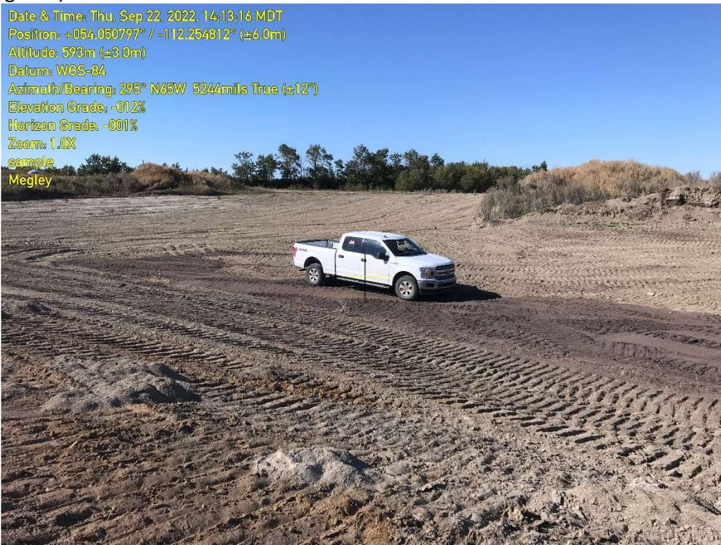
Photo 2: Photo taken looking northwest of the backfilling and recontouring of the dugout (2<sup>nd</sup> waterbody on site).
